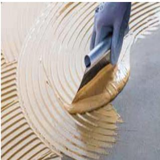
Picture 2. Plank Bonding
